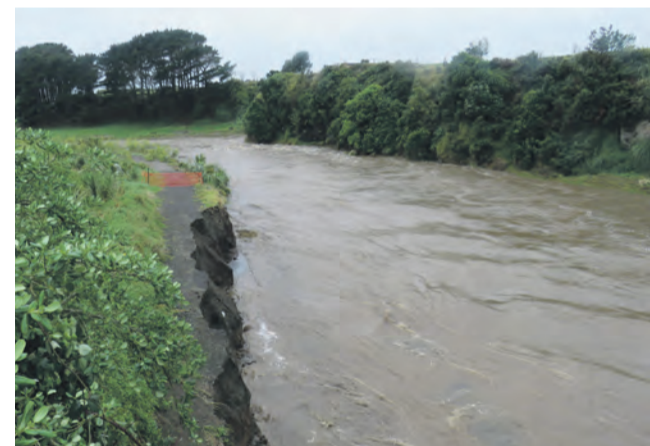
The Waiaua River which scoured out part of the Opunake Walkway at left.
